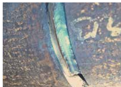
IAC - Vertical downward welding of a root pass in a district heating pipe. Welding speed is significantly increased compared to traditional upward welding.
