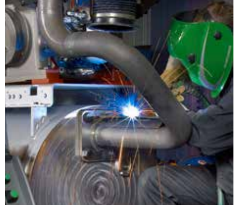
Welding in mild steel.
